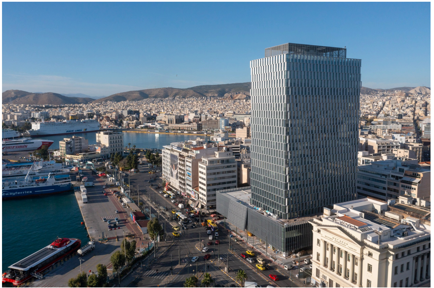
PIRAEUS TOWER, DESIGN BY PILA | Photos ©NikosDaniilidis
