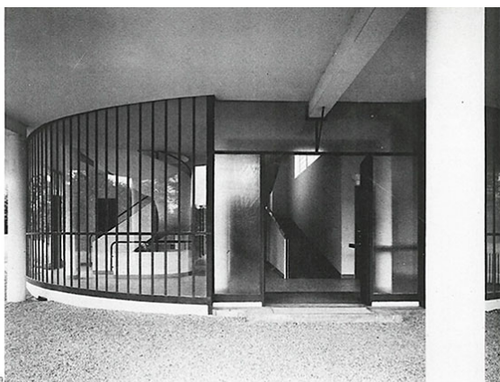
29. Villa Savoye entrance: beam from column in foreground meets beam between columns inside that flank door, thus articulating entry. Straight ahead is the ramp. 30. entrance hall with ramp on right and service stair on left. 31. first-floor terrace, looking away from living room. 32. at head of ramp on first floor looking past service stair towards Madame's bedroom.
